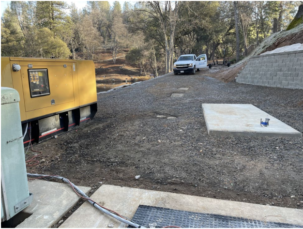
9 - New Concrete Pad LS 13
