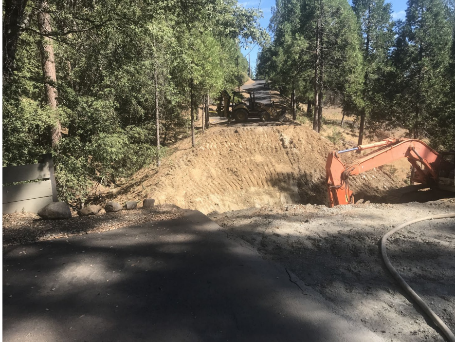
11 - Upper Skyridge Replacement - 30+ Feet Deep
