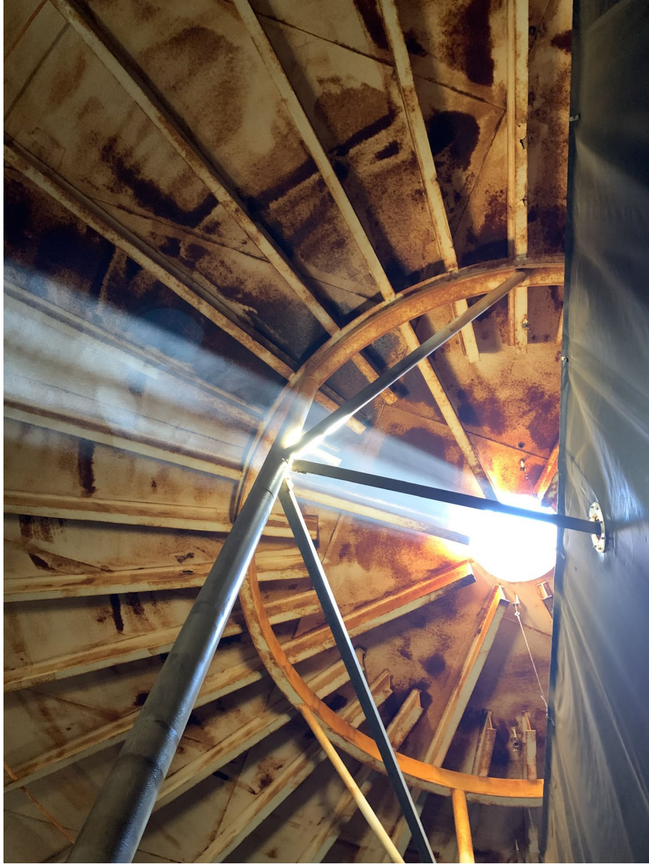
1 - 2G Clearwell Before Sandblasting and Repairs
