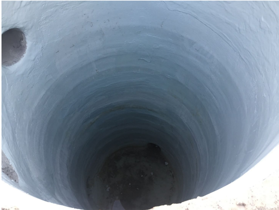
29 - Standpipe Coating to Preserve Concrete
