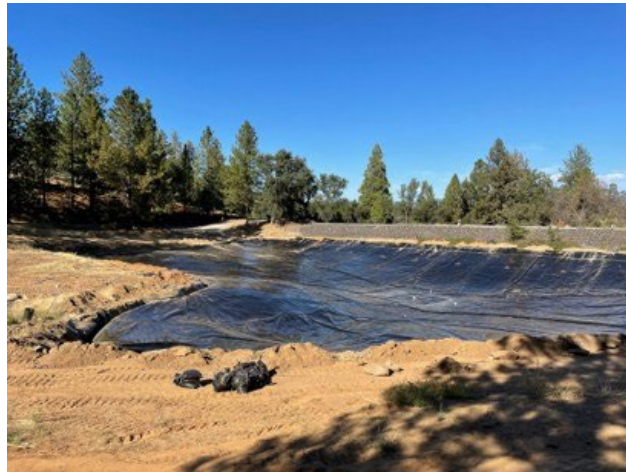
20 - Worn Out Liner Replaced
