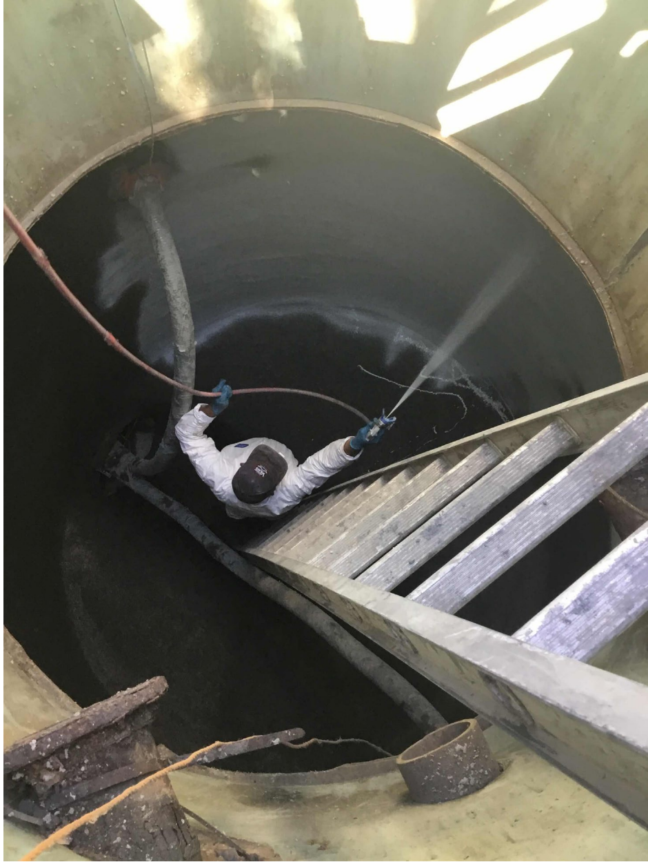
15 - Applied Epoxy Coating to Eliminate Concrete Corrosion
