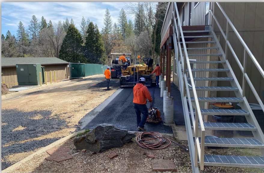
23 - Removed and Replaced Failed Sections of Asphalt
