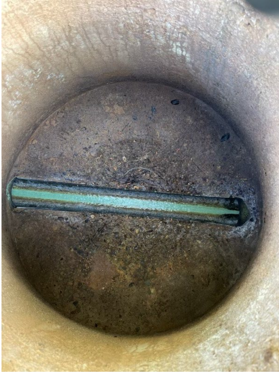
17 - Dozens of Manholes Rehabilitated
