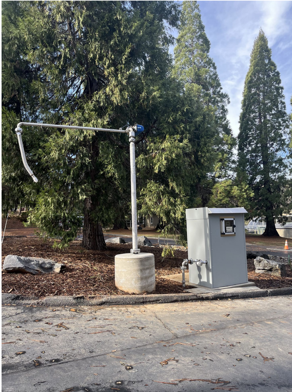
6 - Fill Water Trucks, Tanks and Jugs
