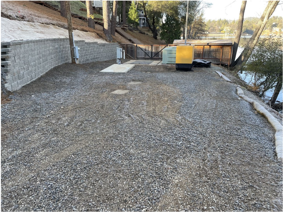
8 - New Retaining Wall at LS 13
