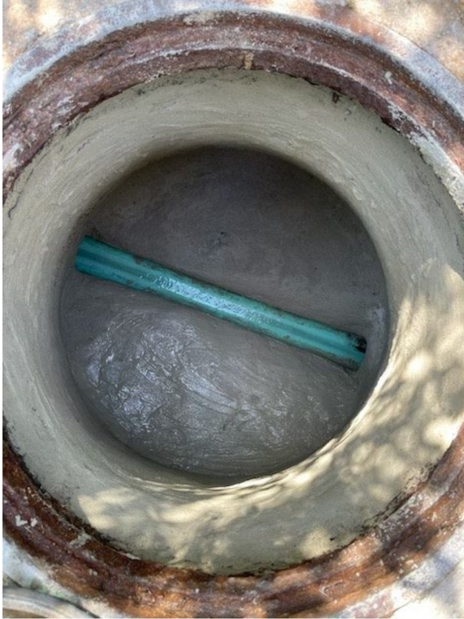
18 - After Manhole Epoxy - Easy Cleaning, Eliminate Leakage (infiltration), Reduce Odors
