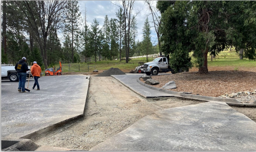
23 - Removed and Replaced Failed Sections of Asphalt
