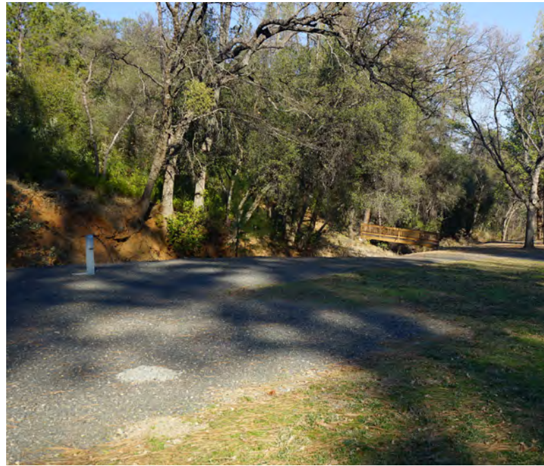
Clean up utility installations.
