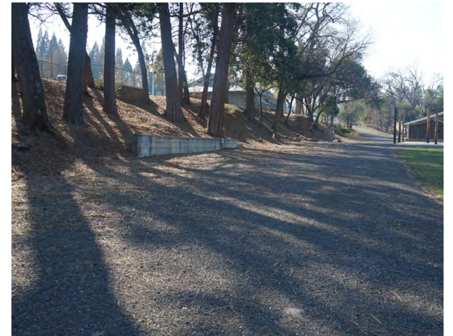
Remove old foundations / abrupt grade changes.
