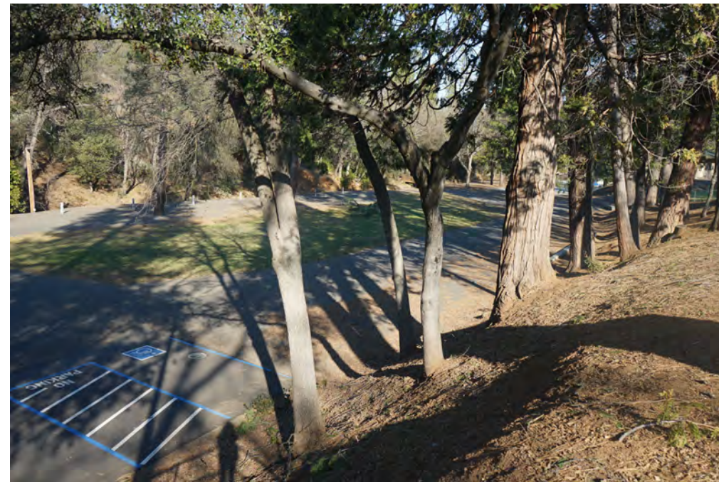
Stabilize eroding steep slopes
